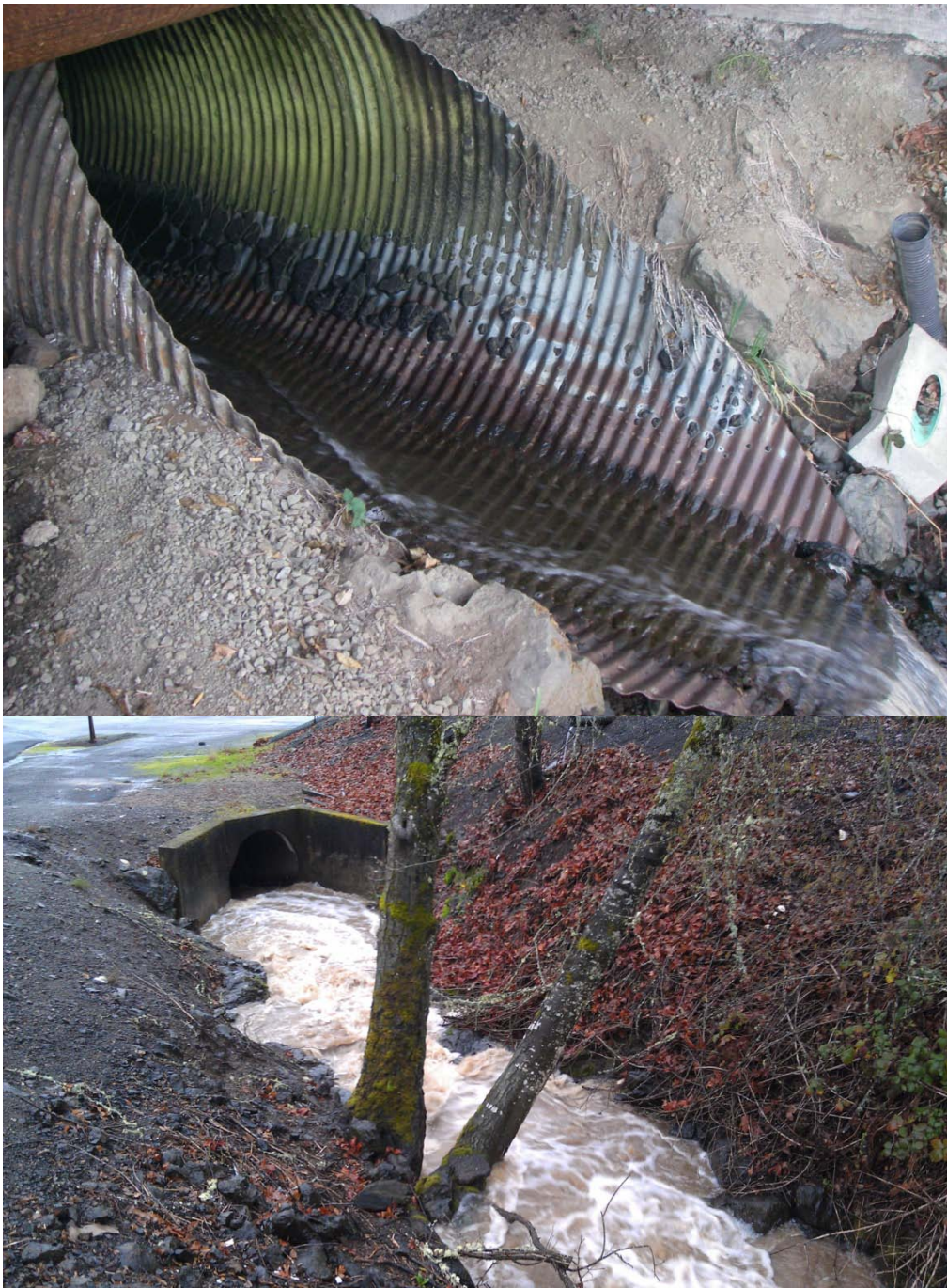
Figure 2. Downstream and upstream of ODOT culvert.
