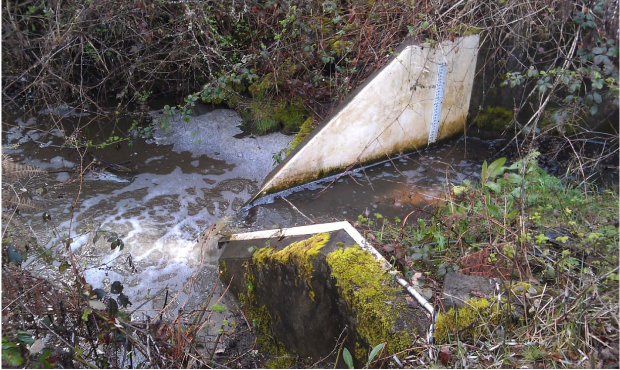
Figure 4. Concrete structure roughly 200ft up from the ODOT culvert.
