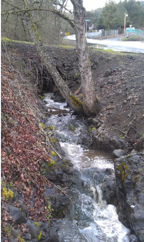
Figure 3. Culvert under Chewaucan Lane 50ft above the ODOT culvert.
